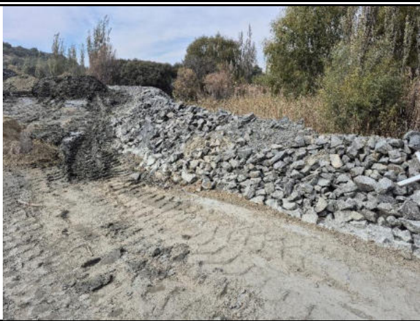
Improved stormwater berm at the southern boundary of the mine
