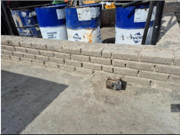
Hazardous waste storage area with locked outlet valve
